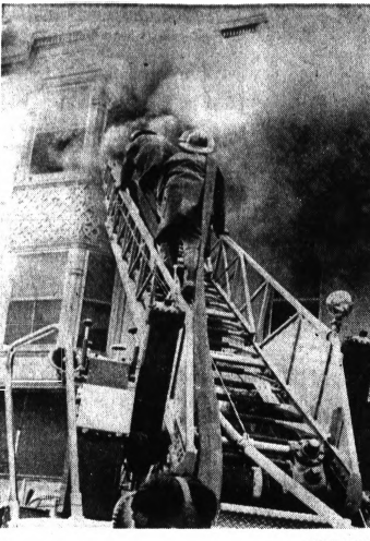
FIRE FATAL TO FIVE — Firemen in Omaha, Neb., climb a ladder to the third floor of the burning Hotel Jackson to fight a blaze and hunt for bodies. The fire, which burned out the top two floors of the three-story hotel yesterday afternoon, killed five and sent four to the hospital.
