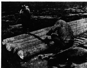
A raft is built from balsa logs, wooden dowels and strips of bark, for the return journey.
