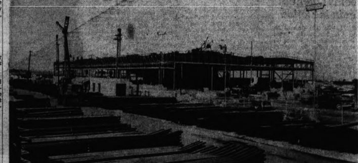
FOR ASSEMBLY OF TRUCK FRAMES — Newest addition to GMC Truck & Coach Division's manufacturing facilities in Pontiac is this 35,000-square-foot truck frame assembly building. Adjacent to GMC's Engine Plant on South Boulevard, the one-level structure will be used for drilling and fabricating frames in readiness for final assembly operations. The structure is scheduled for completion Dec. 15.
