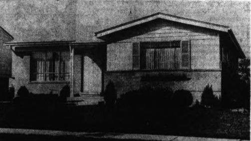
IN MAPLE HEIGHTS — This is the home of the James McKays on Dreen Street in Maple Heights. The exterior is gray brick and white siding. Trim is aqua. The McKays' lot is 50 by
