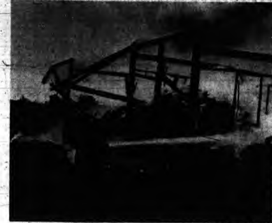
FIRE DESTROYS BARN — Last remnants of the walls begin to collapse as a barn at Van Dyke and 23-Mile roads burned Saturday afternoon. Firemen from the Washington and Romeo fire departments prevented the fire from spreading to nearby buildings. Cause of the fire, which caused an estimated $4,000 damage to the barn and its contents, was undetermined. Owner of the barn was Herman A. Shields, 12350 23-Mile Road.
