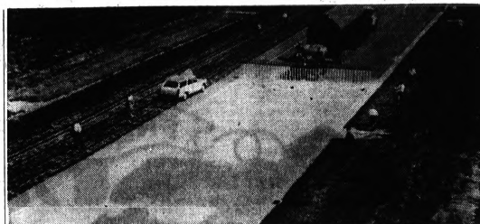
FOAM LANDING STRIP — This truck-trailer spreader at the Toulouse airfield in France puts down a layer of carbonic foam
