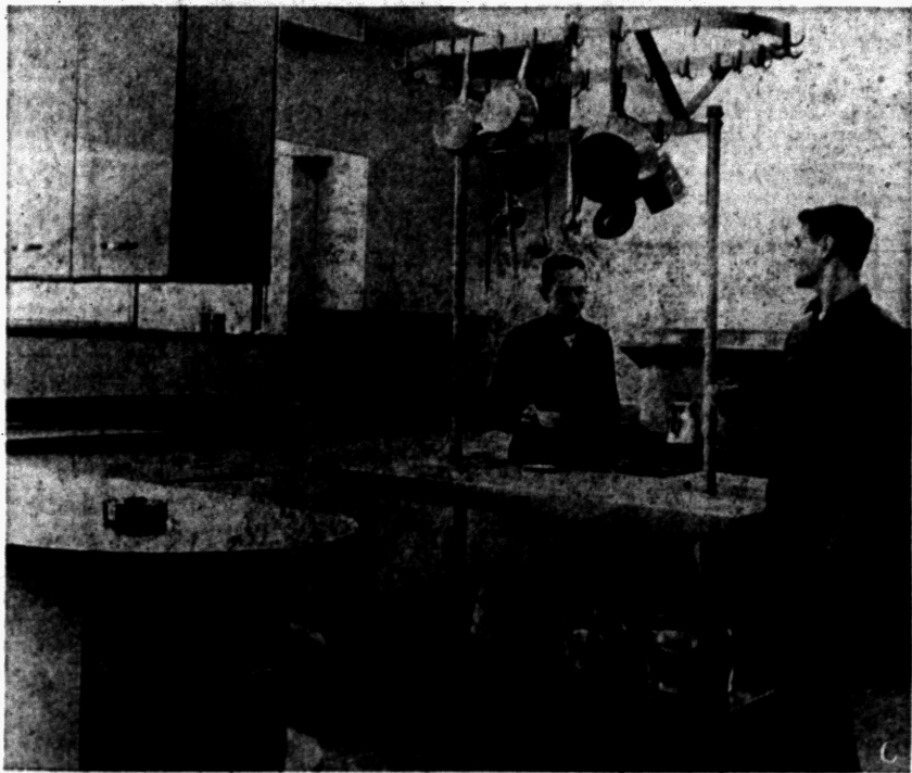
COFFEE TIME IN No. 5 — Firefighters Jerome Lauring, 2133 Mott St., and Grant Hoffmann, 82 Ruth St., try out the kitchen facilities at the new $100,000 Pontiac Fire Station 5, Genesee avenue and W. Huron street, which
