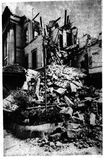
COURTHOUSE CRUMBLES — A historic landmark of downtown Pontiac, the old Oakland County Courthouse, was razed this year when the county no longer had any use for it. Its function had been replaced by the new courthouse in the county service center area. A parking lot now fills the spot at Saginaw Street and Huron Street where the old courthouse once stood.
