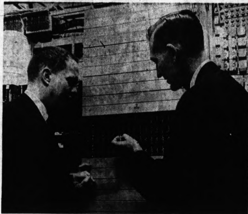
COMPLEX EQUIPMENT—Intricate telephone switching equipment, installed at Pontiac Osteopathic Hospital, is shown to Jack
