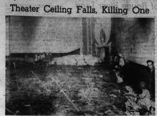
After the Crash —Here's how the inside of a New Orleans movie theater looked Sunday night after the inner ceiling collapsed, dumping a ton of debris on more than 100 movie goers. The falling rubble killed a 65-year-old woman and left 45 others injured. A split-second warning screamed by an unidentified man probably saved the lives of others in the audience. Firemen (right) are looking for victims under the blanket-like debris.
