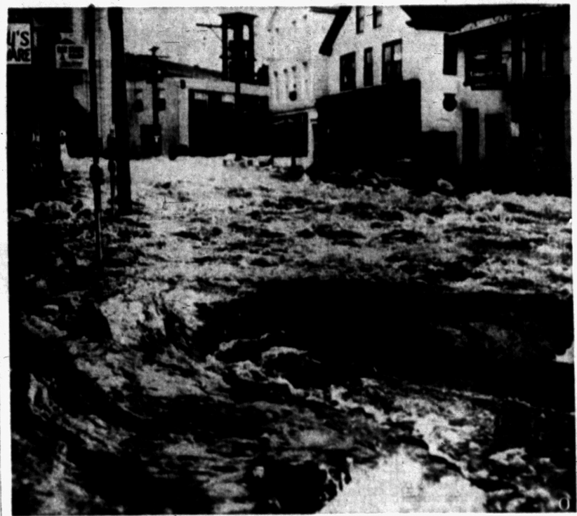
TOO MUCH AT ONE TIME —Water from a broken dam rushes down the business section of Thompsonville, Conn. as a result of the heavy rains. Sidewalks and pavements were swept away by the force of the water.
