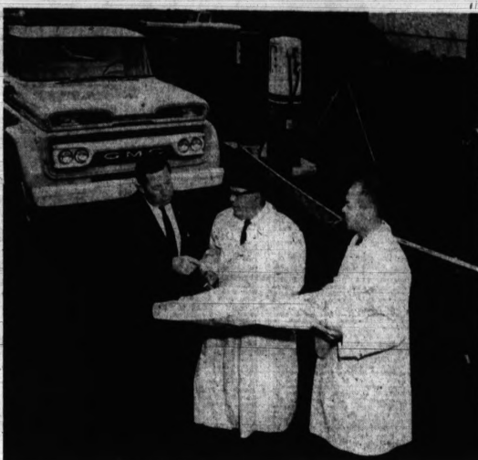
AT GMC SITE — Looking over blueprints with J. S. Davis (left), manager of the GMC Truck & Coach Division Detroit factory branch, are contractor J. A. Fredman (center) and
