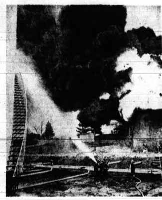
GENESEE OIL TANK FIRE — Firemen are shown wetting down oil storage tanks next to one spewing flames at a Marathon Oil Co. storage area in Genesee Township north of Flint today. The blaze burned itself out after 2½ hours, leaving three firemen injured and more than $30,000 in damage, according to a company spokesman. The tank apparently was set afire by lightning.
