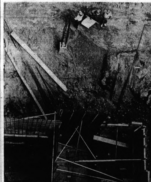
HOSPITAL ADDITION UNDER WAY — If you're going to build a hospital addition, one of the first things you do is lay the foundation for the elevators. This view from the top of Pontiac Osteopathic Hospital shows how the elevator shafts are already in place to serve the two-story addition under construction at the northern end of the seven-story hospital. The addition is to be finished by the fall of next year.
