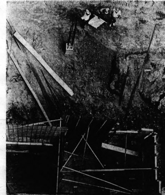
HOSPITAL ADDITION UNDER WAY — If you're going to build a hospital addition, one of the first things you do is lay the foundation for the elevators. This view from the top of Pontiac Osteopathic Hospital shows how the elevator
