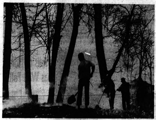
BRUSH FIRE — More than 100 teen-agers and adults turned out yesterday to help clean up the proposed Sylvan Lake Community Center, 2456 Pontiac Drive. The volunteers burned away brush, raked leaves, and spruced up buildings on the site that formerly was a trash air camp. Directed by Dale Hanson, chairman of the steering committee, the residents hope to have the three-acre recreation center ready for summer activities.
