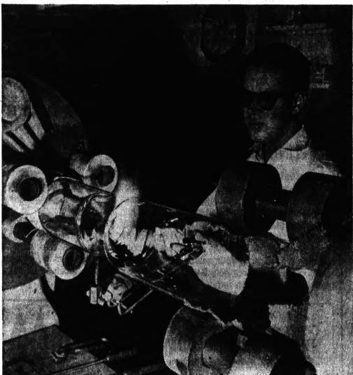
Using lethe and carbon paddle, trainee cuts long glass tube into custom-size container.
