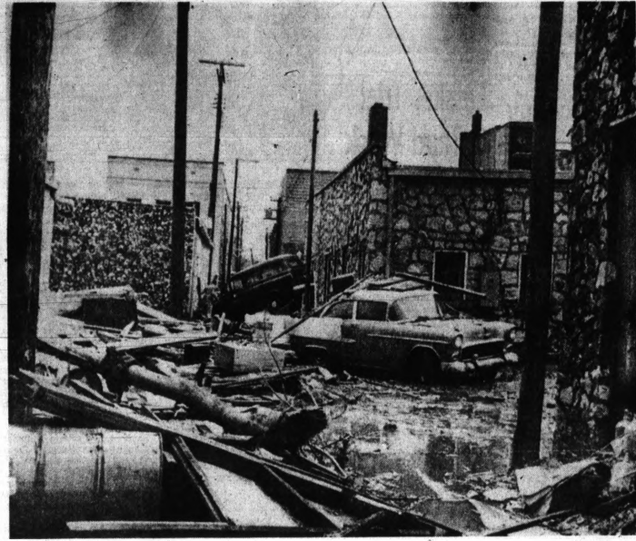
FLOOD CAME BY — Two automobiles rest among wreckage in an alley behind the business district of Harrison, Ark. after a flash flood gurgled through Sunday. Two persons were drowned and an estimated 80 per cent of the business district was heavily damaged. This scene was repeated many times over the weekend as tornadoes and floods struck in wide areas of the Southwest.
