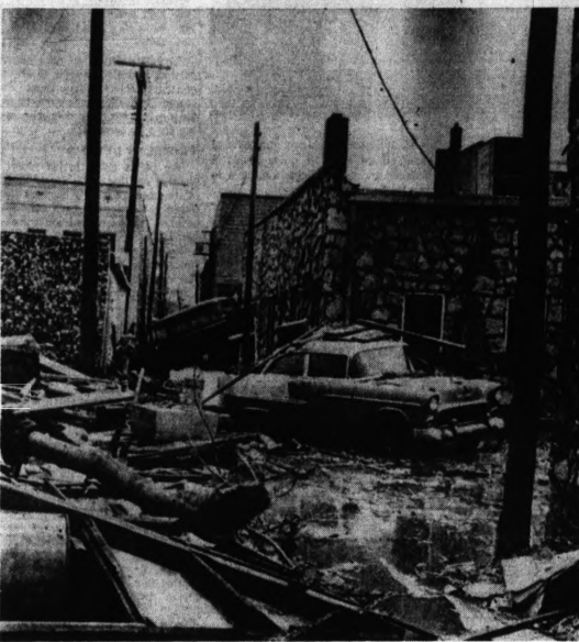
FLOOD CAME BY — Two automobiles rest among wreckage in an alley behind the business district was heavily damaged. This scene was repeated many times over the weekend as tornadoes and floods struck in wide areas of the Southwest.
