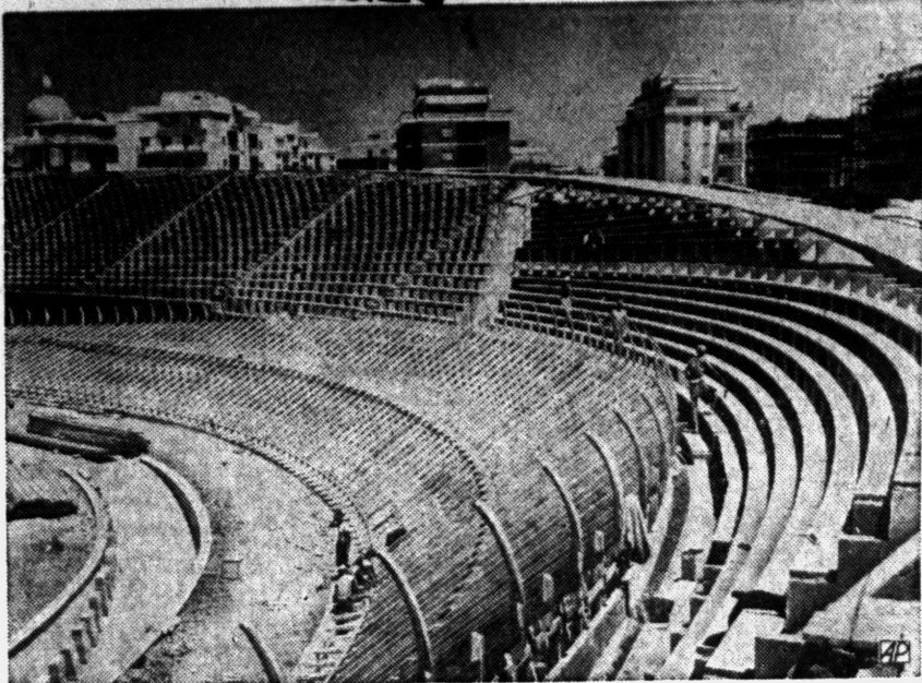
SUMMER CURVE — Foundations for turn construction in Rome, Italy. Cycling events of 1960 Olympics will utilize track.
