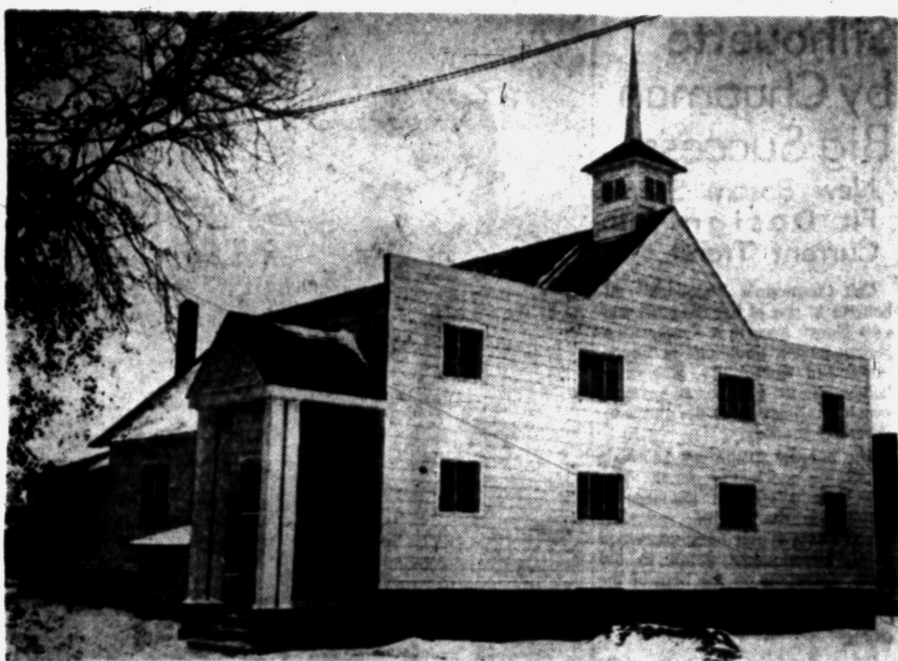
TO BE DEDICATED—A church which grew with the years is Highland Church of the Nazarene, which will be rededicated at a 7:30 p.m. service Tuesday. Originally built in 1921, the church has been remodeled to more than double its capacity.
