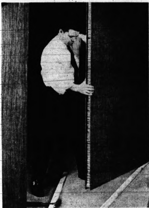
ERECTING JIFFY WALL — "Honeycomb grid" fills the hollow panel of new wood paneling, eliminating an age-old source of noise. Sandwich panel is being positioned here so that bottom edges fit snugly over a 1- by 2-inch base.
