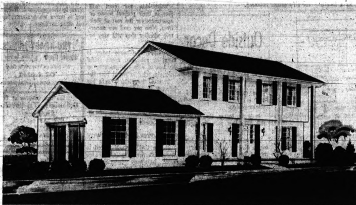
SOUTHERN COLONIAL — More than 400 new homes have been built by the Robertson Brothers Construction Co. in a new subdivision, Hickory Heights on Adams south of Long Lake Road. This "Fox Chase" model sells for $33,400 and features
