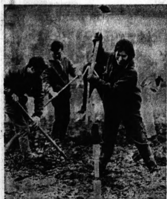
STUDENTS AT WORK — Marcia Aronoff, 20-year-old Oberlin College senior from Middletown, Ohio, drives a stake into the ground in ankle-deep mud prior to the pouring of the foundation of the Antioch Baptist Church at Ripley, Miss. Miss Aronoff is one of 26 Oberlin students rebuilding the Negro church, destroyed by fire after a civil rights rally.
