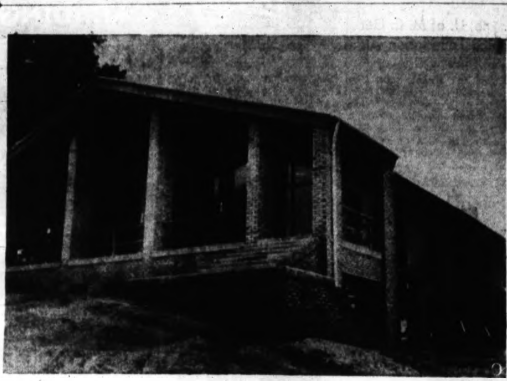
CHURCH OPENS SUNDAY — The new First Church of Christ, Scientist, in Romeo will be open for services Sunday. Visitors also will be welcome to tour the two-story building, on Prospect street at W. Gates street, Sunday afternoon. The new edifice houses a main auditorium on the upper level and a large Sunday School room on the floor below.
