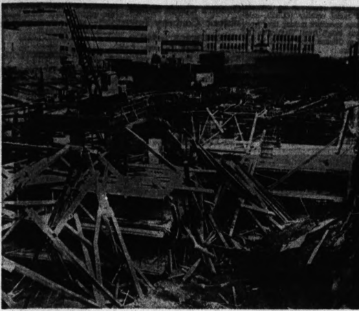
ACCIDENT SCENE — This is how it looked on fashionable Wilshire Boulevard in Beverly Hills, Calif., at the spot where foundation work for a $13.5-million bank building collapsed with a roar, leaving tangled scaffolding and debris
