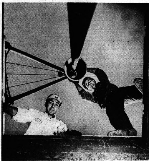
PREPARING FOR WATER — Hopefully awaiting the day when well No. 9 is pumping water again are City Water Department employee Louis Flores (left), of 2986 Pridham, Keego Harbor, and Jim Parker of Layne Northern, a housing well installation company. They have been working on the installation of a new column in the well and repair of existing columns.
