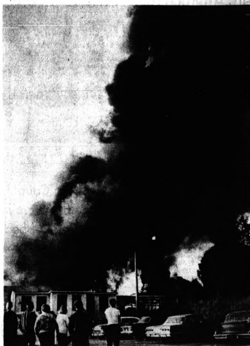
OUT OF CONTROL—A plastics manufacturing factory was hit by an early morning fire that sent huge clouds of black smoke skyward. The flames, started from an oil leak, destroyed the single-story structure.
