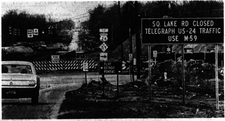
CLOSE ROAD — East-West traffic on Square Lake Road has no road to travel. Square Lake Road is closed while State Highway Department crews widen the road from four to six lanes. Construction of the divided highway is to be complete by Oct. 1. (See story, page A-2.)
