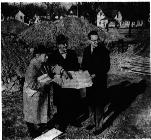
REDEVELOPMENT KICKOFF —City officials paused to formally break ground yesterday for Pontiac's first major urban renewal home building project. Looking over plans are (from left) H. H. Dubbs of Goodell Builders, Inc.; Mayor Robert A. Landry and James L. Bates, planning and urban renewal director. Builders have purchased 23 lots in the R20 project and plan to have three models open by May 1.
