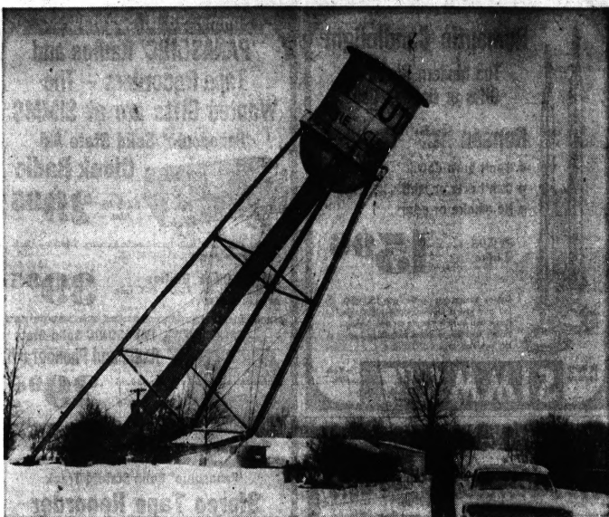
TIMBER-RR —Utica's 40-year-old water tower falls to the ground. Unused for the past three years since the city connected with the Detroit water system, the tower was ordered torn down by city officials. Its only purpose recently was a billboard for graduating seniors who scaled its height to proclaim their prowess to the world. No plans for the water tower site on Auburn near the dump were indicated.
