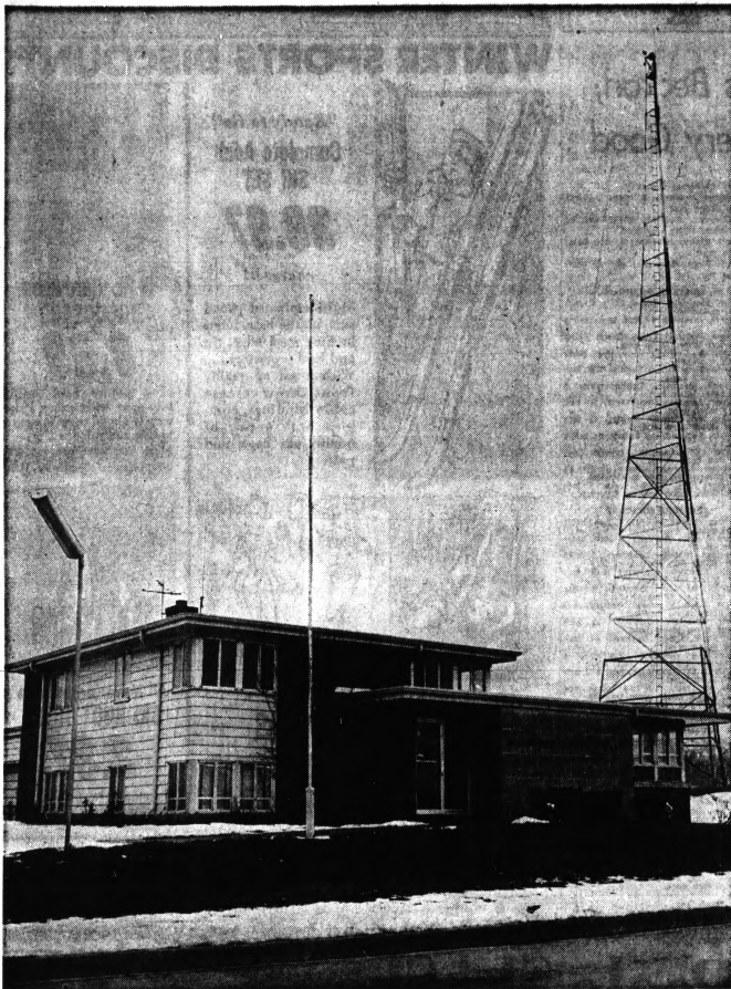
PONTIAC POST — Built less than 10 years ago, the Pontiac post of the Michigan State Police is the work center
