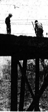
BRIDGE REPAIR STARTED —Workers from the New York Central Railroad began replacing the charred timbers of this wooden bridge on Gunn Road in Oakland Township yesterday. They expected replacement to be complete by today or Monday. The road has been closed between Adams and Orion roads since the July 12 fire caused by sparks from a train passing under the bridge.
