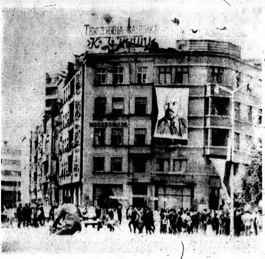
REPORTEDLY LEVELLED — The New Macedonia Hotel in Skopje, Yugoslavia, shown in this view last month, was destroyed and most of its guests killed in an earthquake today.
