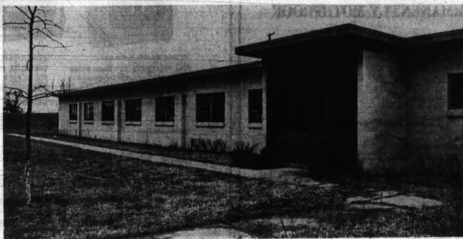
OLD BARRACKS, NEW USE? — This building housed soldiers a few years ago when the U.S. Army was operating a Nike anti-aircraft missile base near Auburn Heights. Now,
