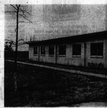
OLD BARRACKS, NEW USE? — This building housed soldiers a few years ago when the U.S. Army was operating a Nike anti-aircraft missile base near Auburn Heights. Now,
