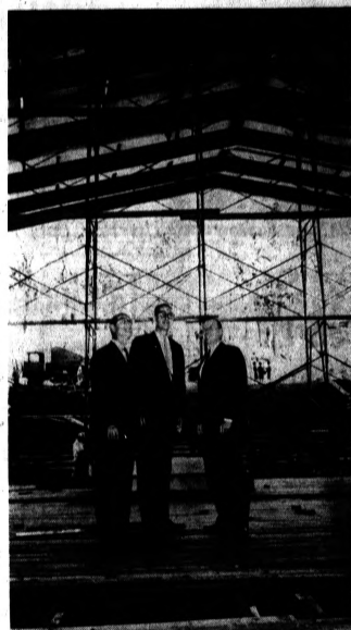
IT'S TERRIFIC — Ken Morris, codirector of UAW Region 1 (left); D. B. Varner, chancellor of Oakland University (center) and UAW President Walter P. Reuther check on the progress made in building the Howard C. Baldwin pavilion for the Meadow Brook Music Festival.
