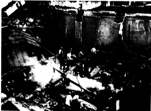
SUPERMARKET WRECKED — Firemen search the wreckage of a Brooklyn, N.Y., supermarket after the roof collapsed, wrecking the two-story building yesterday afternoon. There were no known fatalities, but 23 were injured. About 50 persons were inside when the roof fell in. (See story, page A-2).
