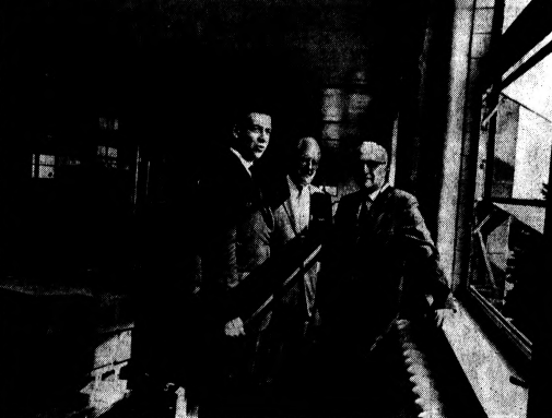
VISIT COLLEGE — John E. Tirrell, president of the Oakland Community College (left) yesterday escorted two county physicians around the Highland Lakes campus at the former TB sanatorium, now undergoing extensive remodeling. The doctors, Dr. Frank J. Condon (center), deputy director of the county health department, and Dr. William F. Fidler, TB control officer of the department, were invited to the campus to dispel rumors that the building is not safe to the health of students.
