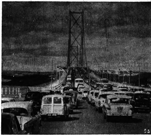
PLENTY OF BUSINESS — Vehicles in rank move across the newly-opened Ford span suspension bridge in the world and the longest in Europe, links Fife and Lothian.
