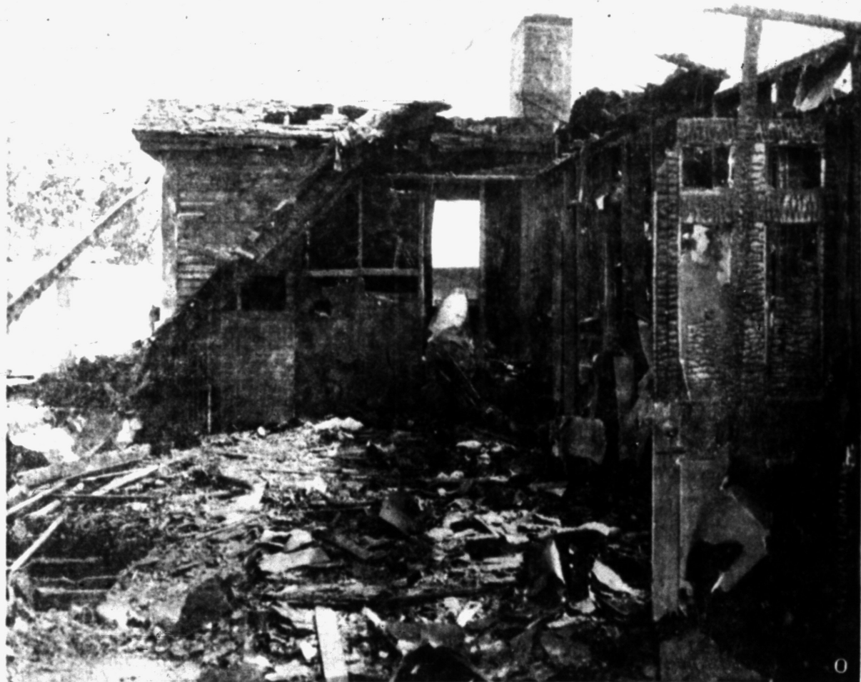
DAMAGED SECTION —Shown above is part of the estimated $500,000 damage caused by the fire, which authorities believe was started by a workman who was burning paint off the hospital with a blow torch. Damage was confined to the upper portion of the 2½-story building. Quick action on the part of hospital attendants led to the rescue of all patients without fatality.
