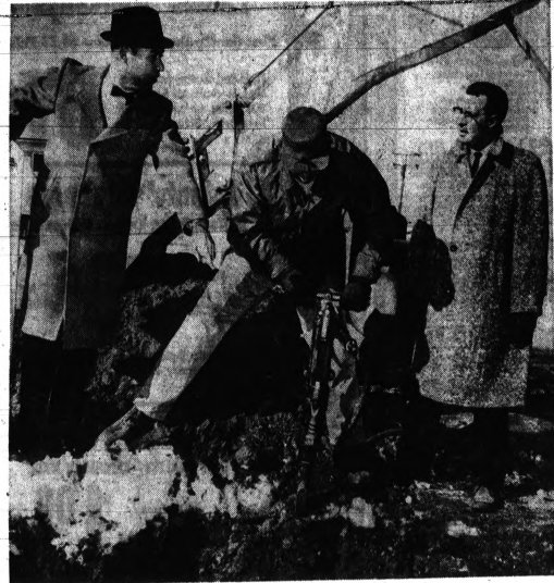
FRIGID WEATHER BYPRODUCT—Looking on as Bill Wilson, Independence Township water superintendent, uses an air hammer to break the frozen earth are Township Clerk Howard Altman (left), and Township Supervisor Duane Hursfall. Township personnel have already uncovered 54 frozen water lines this winter.
