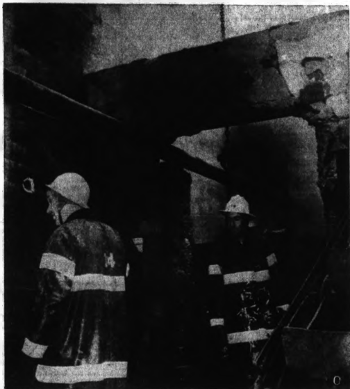
EXAMINE RUINS — Two Oxford firemen survey the damage caused this morning when fire gutted the interior of the Pontiac Hide Co. plant, 885 Lakeville Rd., Oxford. Also on hand to fight the $100,000 blaze were firefighters from Addison and Orion Townships. An electrical spark which ignited naphtha solvent in a storage tank, is believed to have caused the fire.
