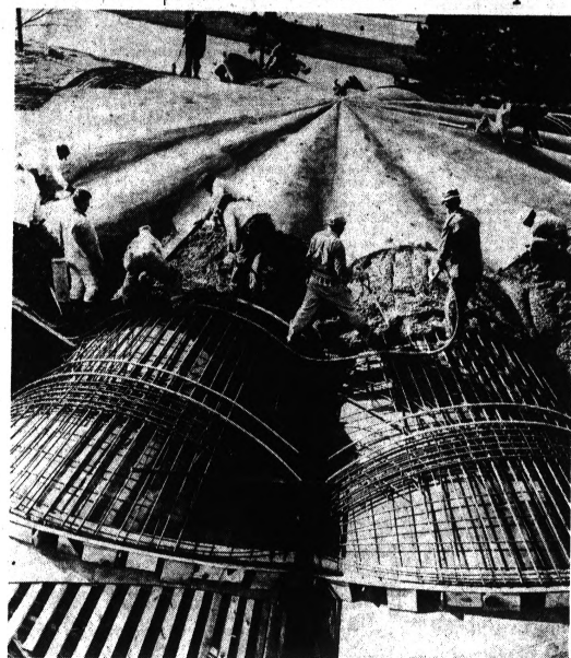
ROOF-POURING PARTY — Officials and friends of the GMTC Employees Federal Credit Union yesterday held one of the most unique parties in history. They had soft drinks and doughnuts while they watched a group of workmen pour and spread 150 tons of concrete to form the roof of the modern circular wing of the new $400,000 credit union building on Woodward avenue across from St. Joseph Mercy Hospital. When finished the roof, with a 60-foot diameter, had a thickness of 4 inches. The entire building is scheduled for completion in January.
