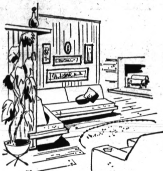
CONVERSATION CORNER — Charming nook in this living room was created by building a banquette seat into one corner. Seat is cantilevered out from wall and built of Douglas fir lumber. Cushions were custom-made to fit. Wall is paneled in autumn-hued western red cedar.
