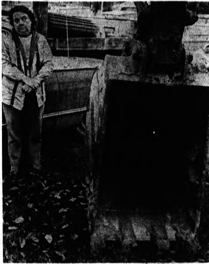
LOOKING IT OVER—Mrs. Wilfred Cole of 914 N. State in Davison held up construction of a sewer line across her property for awhile yesterday by driving her car into the excavation area.
