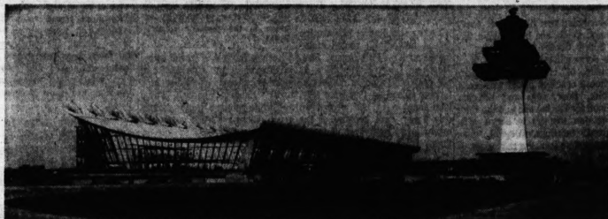
Terminal And Control Tower Designed By Late Eero Saarinen of Bloomfield Hills
