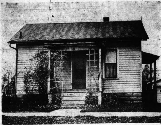
"ROTTEN APPLE" — Although structurally sound, this house at 60 Parkhurst St. was referred to by urban renewal officers as "a rotten apple in a pretty good block." Marked
