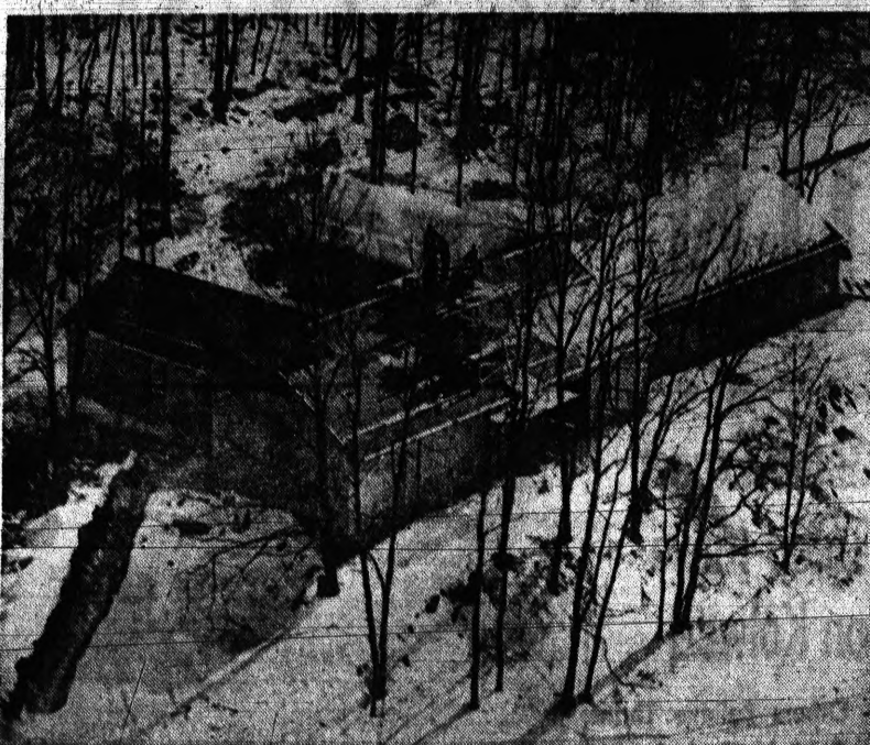
KENNEDY'S NEW HOME — Work goes forward despite snowy weather on President and Mrs. Kennedy's ranch-style house. It stands on Rattlesnake Mountain in the Virginia hunt country near Middleburg. Workmen on a raised platform are putting up a chimney. The house's exterior will be finished in masonry and stucco.
