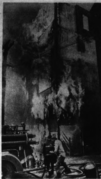
BATTLE BLAZE — Flames leap through the porches of a business tenement building at Main and Springs streets in Holyoke, Mass., Friday as fire fighters prepare to get a hose turned onto the flames. The building has apartments on the three upper floors and a shoe store on the first floor. The fire was contained to a back porch area and one person was rescued from the fourth floor.
