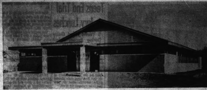
FRIENDLY GENERAL BAPTIST CHURCH —Members of the Friendly General Baptist Church will celebrate the opening of their new church, 69 S. Astor St., tomorrow. Constructed of cinder block, the building is faced with Roman pattern quick brick of a buff color. Valued at $75,000 the new church is located on a lot 130 by 330 feet. The architect was W. B. Edwards of Pleasant Ridge and Robert Fitzpatrick, the builder. Rev. Robert Garner is pastor.
