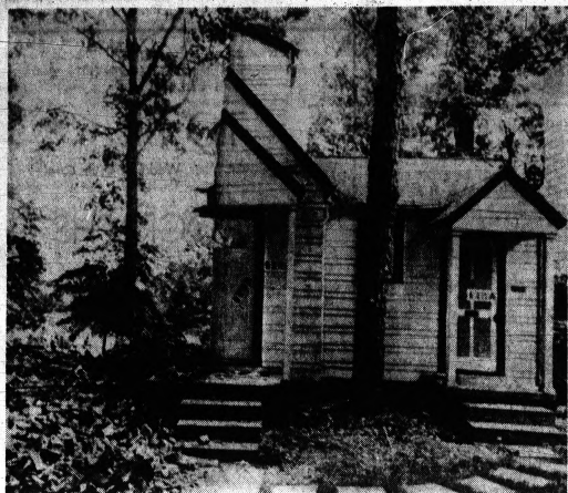
HALF A HOUSE—This is what Joe Conrad has left of his house in Charlotte, N. C., after wrecking crews cleared away the city's half in a move to clear the way for a new street. Joe says he'll remodel and put in office space.
