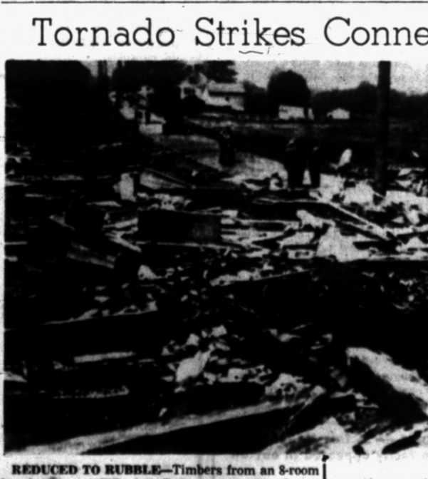
REDUCED TO RUBBLE—Timbers from an 8-room farmhouse near Ellington, Conn. were scattered over a wide area when a sudden tornado hit the area. Two occupants, a mother and son, were found severely injured in an open field after being blown across the highway. A barn nearby also was flattened.
