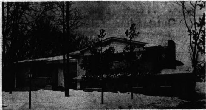
IN SAGAMORE ESTATES — The Leonard Millers built this grayish white brick home on Arrowhead Road about 18 months ago. Fred Horner, AIA, of Highland Park was the architect. Austin Building Company did the construction work. Shutters and iron
