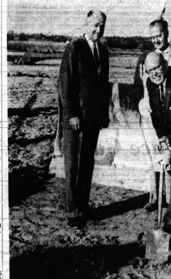
BREAK GROUND—Stanley S. Kresge, president of the Kresge Foundation, breaks ground for the new $1.5 million Kresge Library on the campus of Michigan State University Oakland. The library is being built with a gift from the Foundation. Behind Kresge are
