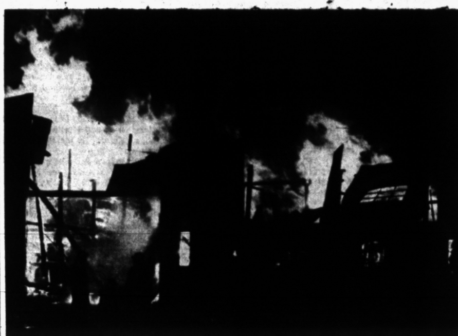
ROOF COLLAPSES—Picture taken above shows building Saturday night, after the roof had fallen. raging fire in the Benson Lumber Co. storage. The building was filled with finished lumber.
