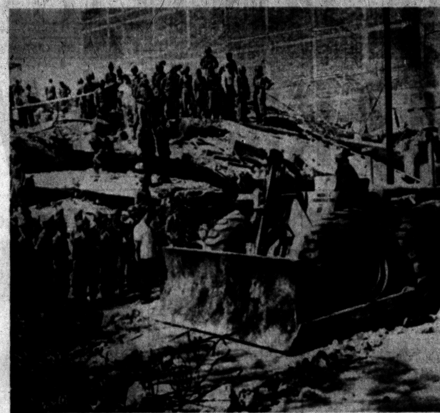
BULLDOZING FOR BODIES — Bulldozers were utilized to search for victims of yesterday's Mexico City earthquake. An estimated 10 persons were believed killed in the collapse of this apartment building. Soldiers in steel helmets aided police and firemen in the grim search.
