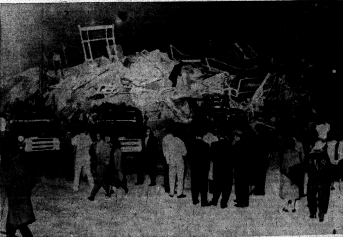
PILE OF RUBBLE — This is what was left of a five-story apartment house following a pre-dawn earthquake in Mexico City yesterday. Four persons reportedly died in this building and many
