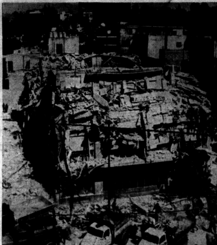
QUASHED IN QUAKE—This four-story apartment was squashed almost flat in yesterday's earthquake in Mexico City. Rubble at the left in picture covers a dozen parking lot. Five persons were believed trapped in the building wreckage.
