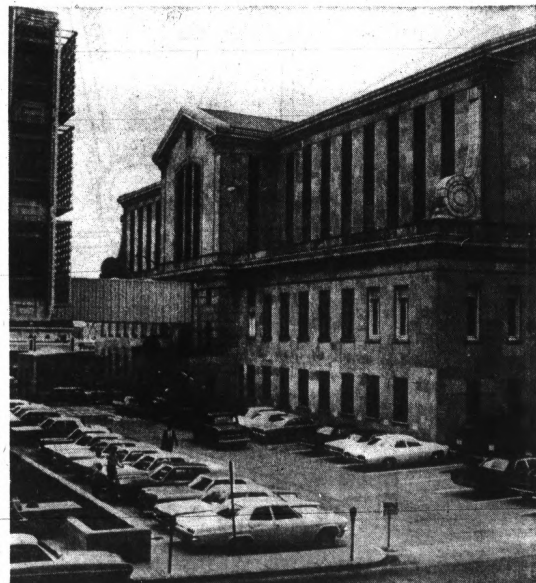
WHERE RAY WILL BE HOUSED —Tight security measures are in effect as the Shelby County Jail, Memphis, Tenn., waits in preparation for the return of James Earl Ray
