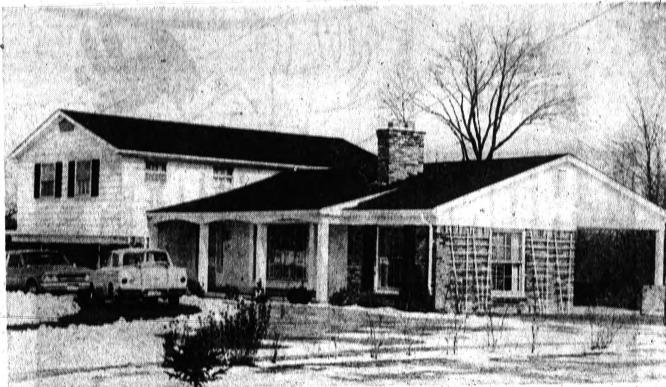
WILCOX HOME —The brick and clapboard trilevel of the Edmund H. Wilcoxes on Thornbriar Way is situated on a corner hill site. Three cars and two car-driving sons, Larry and Tim, could create quite a traffic problem. The fore-
