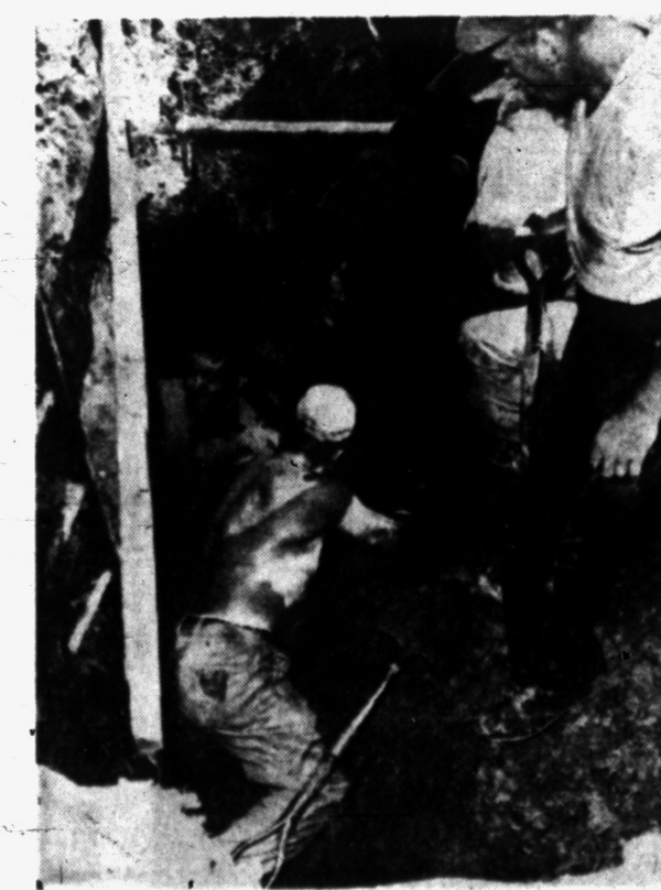
BURIED BY SAND — Romeo Chretien (left) 50, of Lawrence, Mass., was rescued by the efforts of his fellow construction workers after he was buried in eight feet of sand during a sewer trench cave-in yesterday. Friends dug frantically with their hands to free Chretien, after two other men, buried to their waists, managed to dig a hole to Chretien's head and free him. The victim was taken to a hospital suffering from shock.
